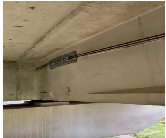
(b) Site inspection photo after 2 years of operation
