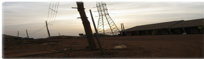
Figure 3. High Tension Cables over a Plot
