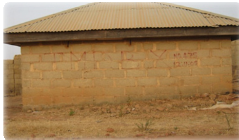
Figure 2. Marking the Structures with Red “X”
