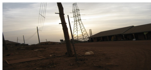
Figure 1. High Tension Cable Passing Over Plot
