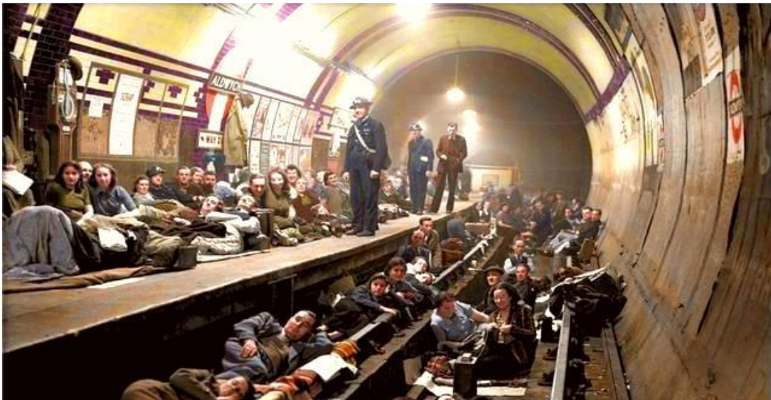
Figure 4. Subway Station Used as an Emergency Shelter for Personnel Protection
