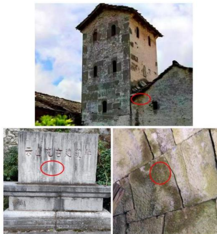
Figure 1. The Current Status of Biological Degradation in Yunfeng Tunpu is Marked as Aesthetic Damage and Stone Damage
