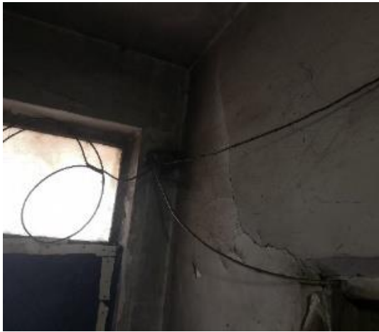
Figure 5. Interior Wall Cracks
