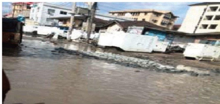
Figure 6. Flooding as a Result of Indiscriminate
