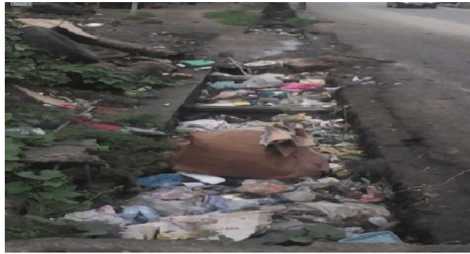
Figure 5. Blockage of Drainage with Solid Market
